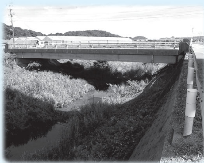
枝橋外橋梁修繕工事
